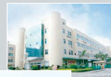
Electric Products Plant, Huizhou
